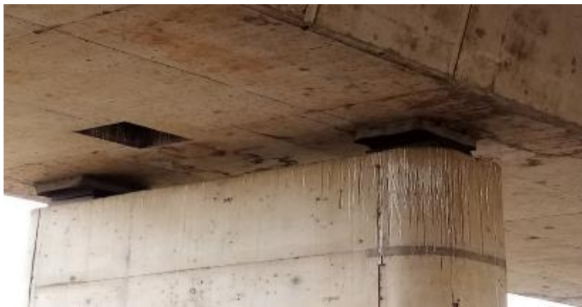
Plate 13 Showing bearings of the Itobe Bridge
