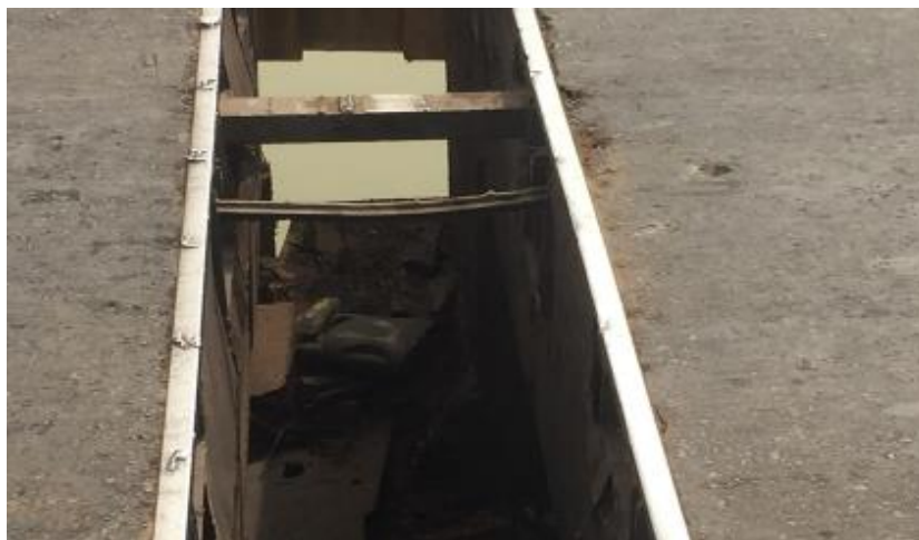
Plate 25 Showing opening of expansion joint
