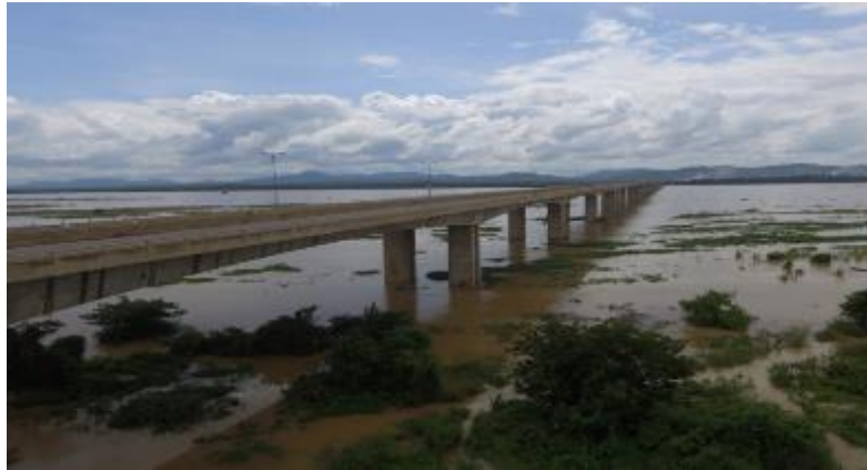
Plate 3 Drone imagery showing side view of Itohe Bridge
