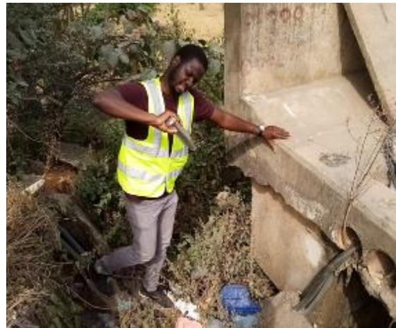
Plate 6 Concrete strength test using rebound hammer device on Bridge Abutment
