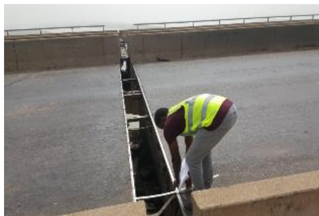
Plate 4 Measurement of exposed expansion joint
