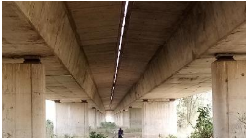
Plate 12 Drone captured images showing bearings of the Itobe Bridge
