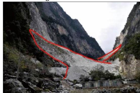
Figure 8 Unstable slopes H4 and H5
