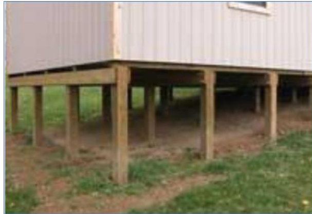
Figure 1 Sloping ground with unequal storey height
