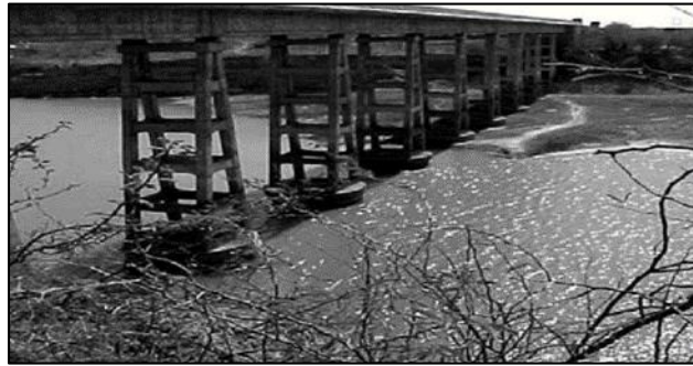
Figure 5 The Rudramata Bridge
