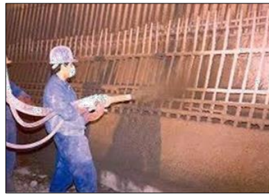
Figure 3 Air form kits, Polyurethane foam and Reinforcing Steel
