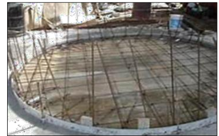
Figure 3 Air form kits, Polyurethane foam and Reinforcing Steel
