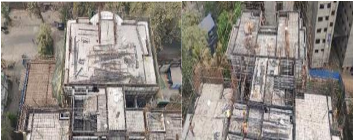
Figure 9 Conventional Shuttering
