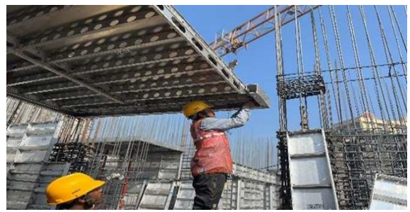
Figure 4 Fixing of deck panel
