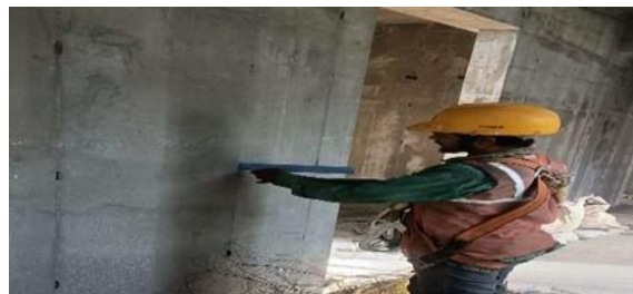
Figure 5 Removing wall tie
