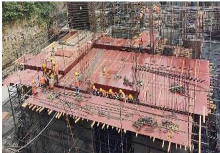
Figure 8 Conventional Shuttering Conventional
