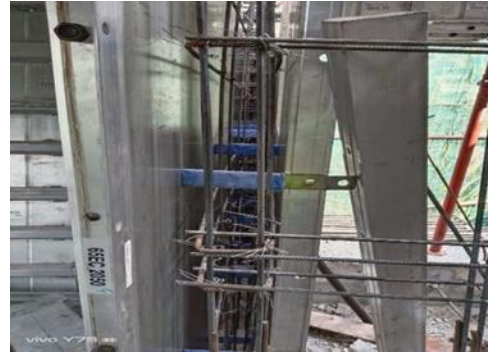
Figure 2 Fixing of wall panel
