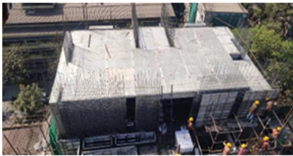
Figure 3 Slab decking
