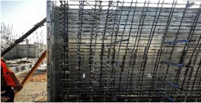
Figure 1 Erection of wall panel
