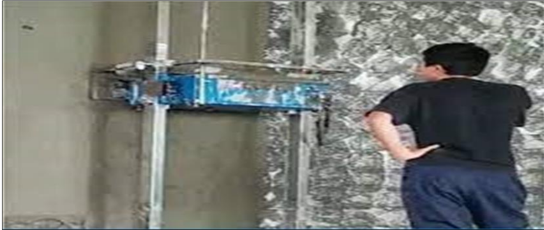
Figure 6 Concrete plastering robot
