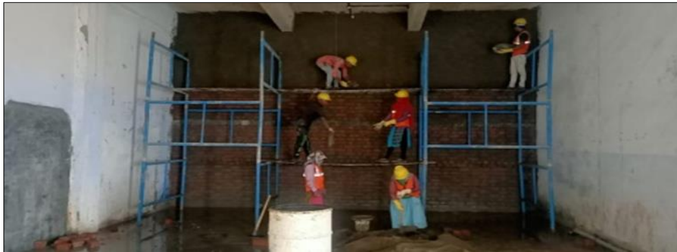
Figure 2 Image of Brick masonry
