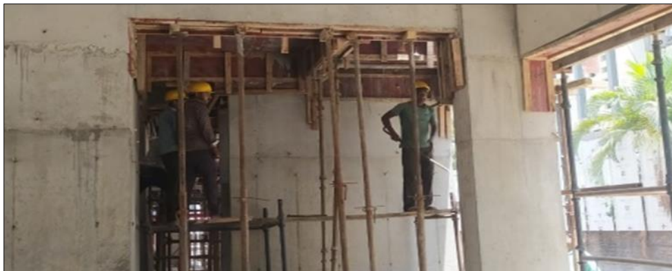
Figure 3 Image of Scaffolding
