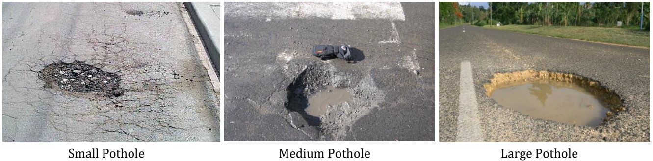
Figure 1 Photos of Different Severity of Potholes
