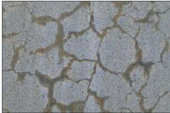
Figure 9 Cracks caused by alkali-silica reaction
