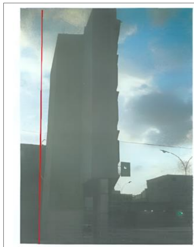
Figure 3 General view of the building after tilt
