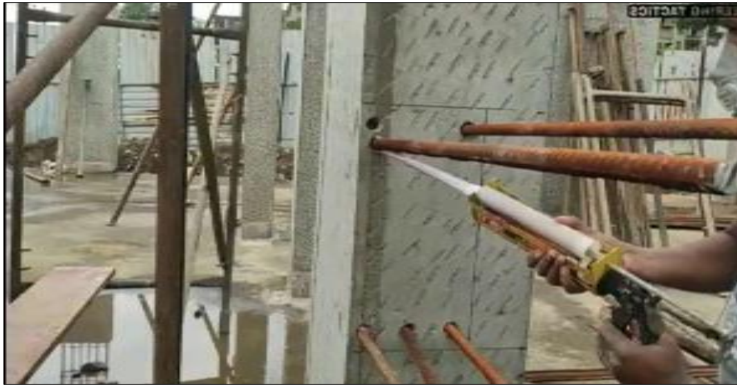
Figure 7 Sample of Column Drilled to Insert New Be
