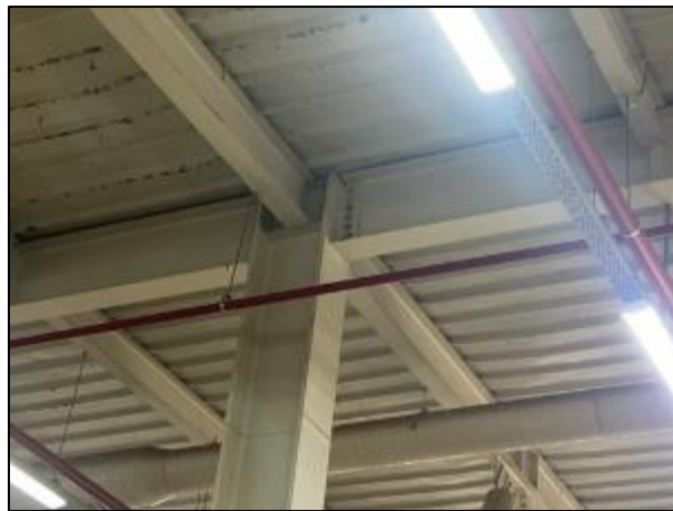
Figure 5 Photographic evidence of weak steel beam–column connection and associated diaphragm separation
