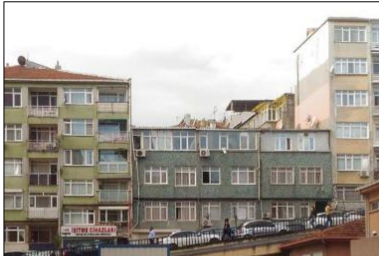
Figure 10 Visual evidence of inadequate seismic gap between two adjacent, dissimilar structures
