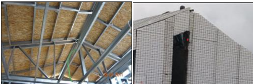
Figure 2 Schematic of a proposed lightweight, engineered CFS (a) or 3D panel roof system (b)
