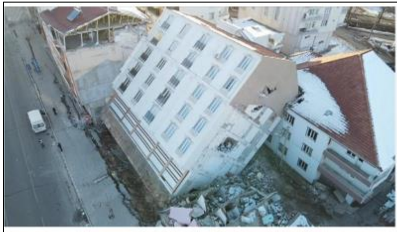
Figure 9 Building collapses caused by soil liquefaction during the February 2023 Kahraman Maras, Turkey earthquake.[13]
