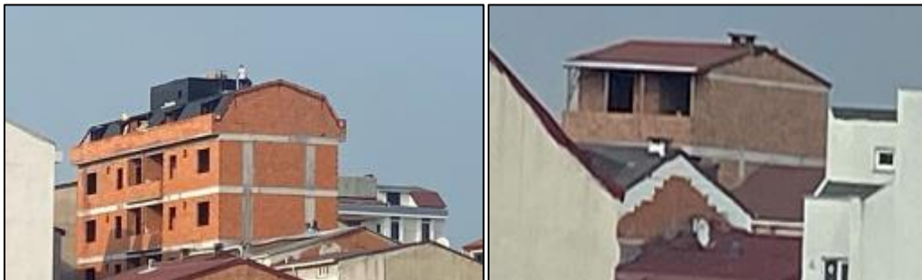
Figure 1 Illustration of non-engineered, heavy roof construction vulnerable to seismic forces
