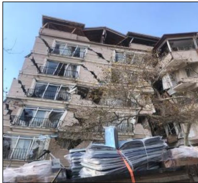
Figure 3 Post-earthquake failure illustrating the collapse of unbraced brick partitions
