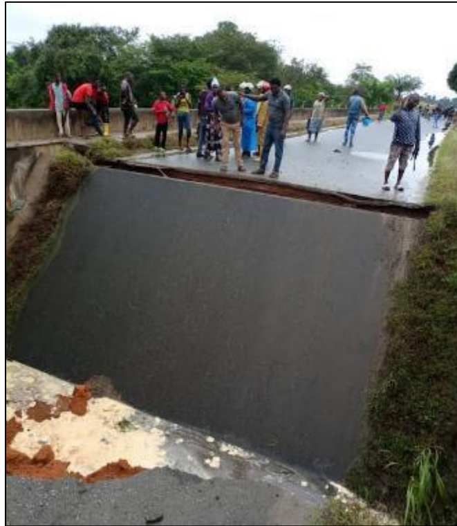
Figure 6 Collapsed link bridge in Delta State
